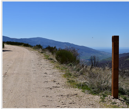
RUTA R06 R06B - SIGN Signpost 55 metres
